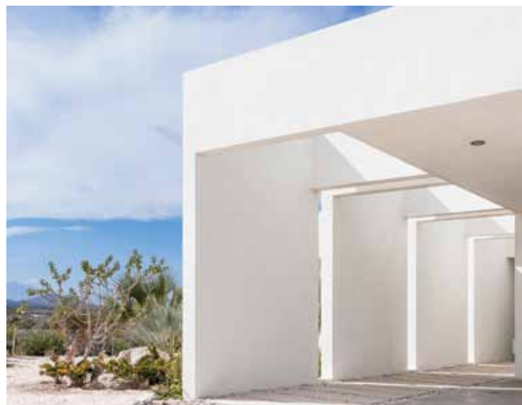
ABOVE AND OPPOSITE: Functional elements of passive ventilation and solar gain are brilliantly integrated into the modern design of House Three. A series of concrete-reinforced insulation panels are artfully arranged to look like a streamlined sculpture—but they act like a smart passive-building system. Two families share the 3,800-square-foot house, sited on about an acre of land.
